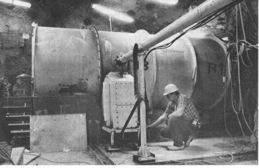
WHERE IT BEGINS — A nuclear device will be placed inside the end of this line-of-sight pipe; radiation will travel down the pipe to experiments located hundreds or thousands of feet away. Mike Burke (9324, seen here) is assistant project leader for the test.
